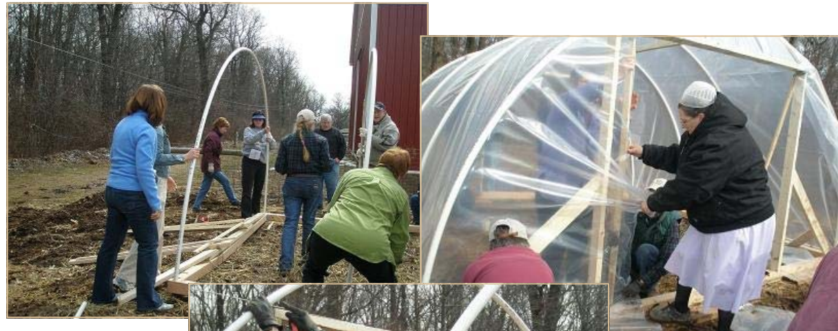
Hoophouse construction at Flint Hill Farm. Photographs courtesy of Anita Russo
