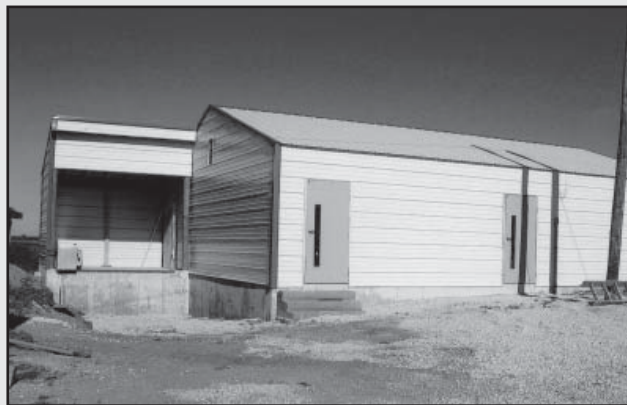
New Century Farm’s new egg processing and storage building under construction.
