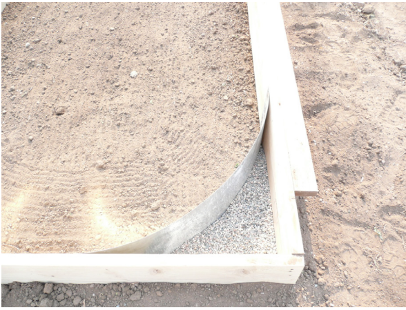
A completed corner.
