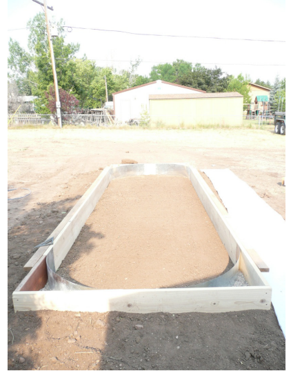
With all four corners finished.
