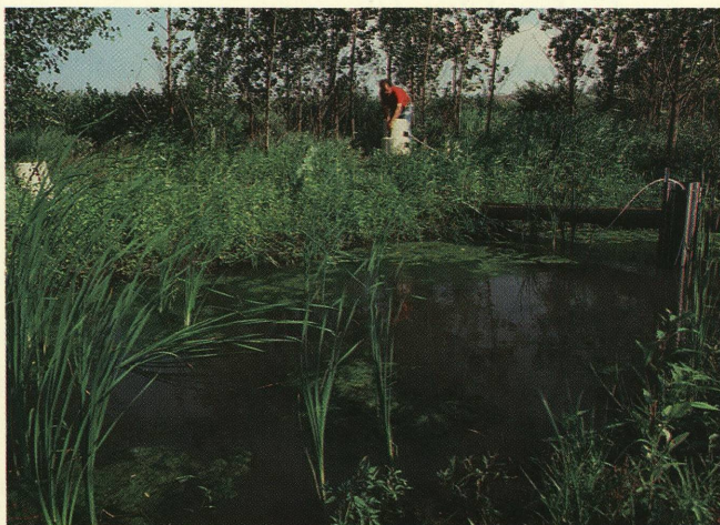
This three-year-old wetland was constructed at a field tile outlet along Bear Creek in central Iowa.
