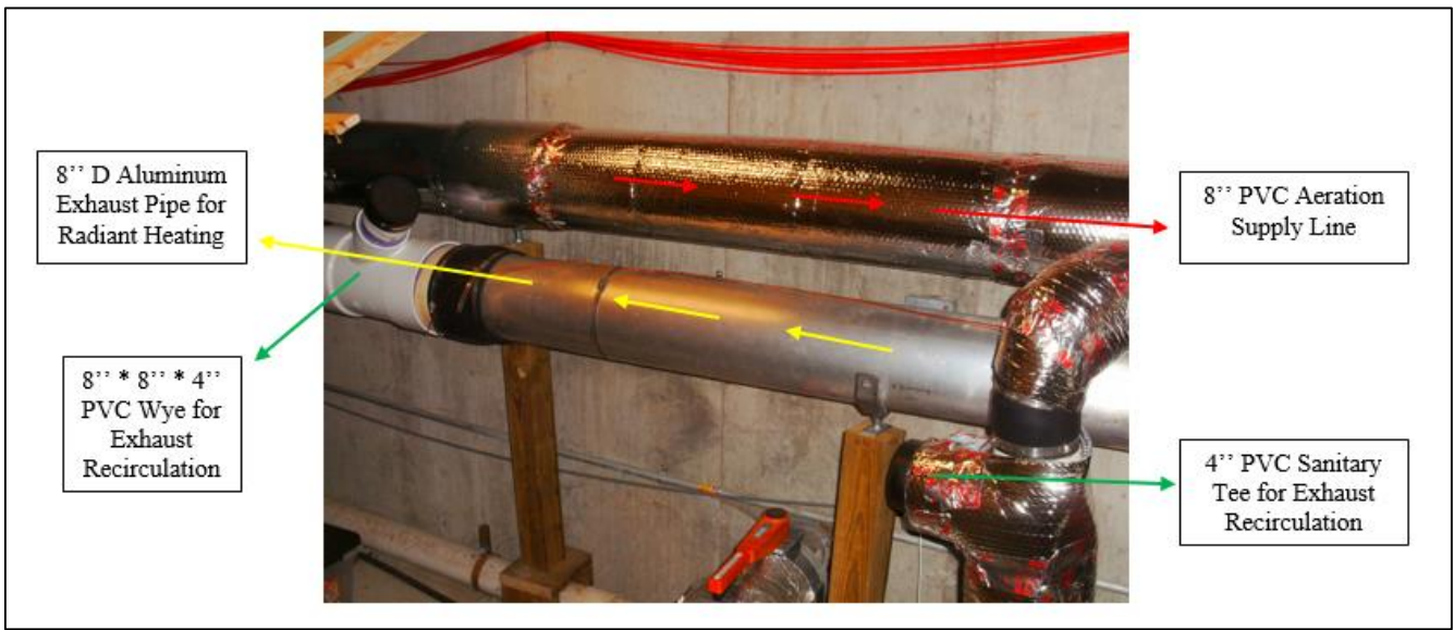
Figure 44: Exhaust Vapor Recirculation Connection Points
