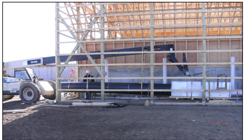
Figure 48: Delivery of Agrilab Technologies Heat Exchange Unit
