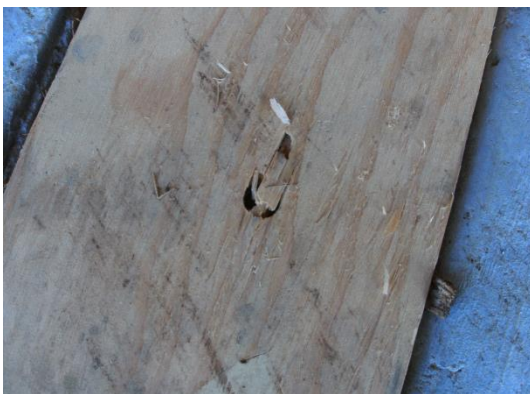
Figure 37: Aeration Hole with Chipping
