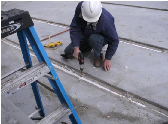
Figure 32: Drilling of Aeration Holes
