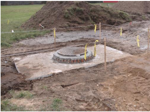
Figure 12: Compost Leachate Tank at UNH Facility
