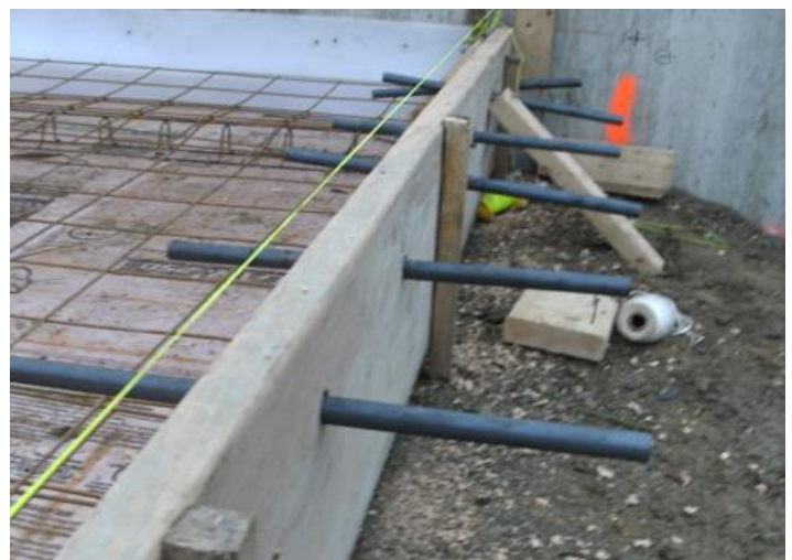
Figure 22: Concrete Slab-Connecting Dowels at UNH Composting Facility
