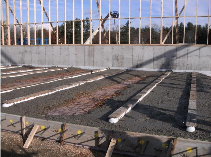
Figure 30: Concrete Pour for Main Composting Floor
