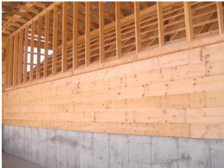
Figure 17: Back Push Wall at UNH Composting Facility
