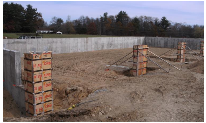
Figure 14: Concrete Piers at the UNH Composting Facility
