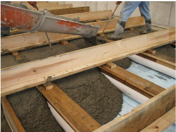
Figure 29: Alternate Cover Plate Form Setup
