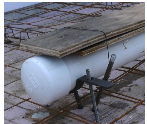
Figure 26: Aeration Line Forms for Cover Plates
