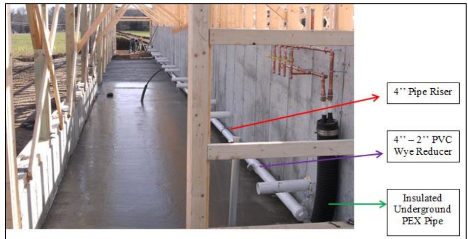
Figure 40: Specifications when Pouring Back Mechanical Floor
