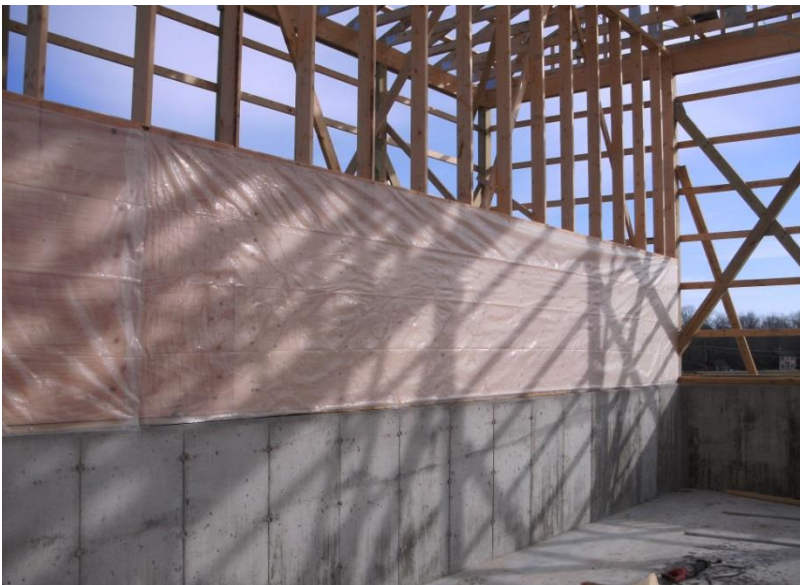
Figure 18: Vapor Barrier on Back Push Wall at UNH Composting Facility
