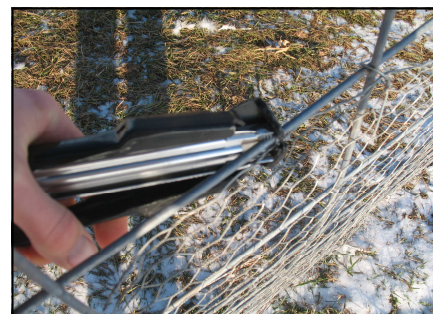
▲ Photo 3. The bottom 3-4 feet of the entire hoopie is covered with 1" chicken wire and fastened to the panels using wire or hog rings.
