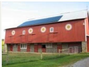
Solar panels, on the south-facing roof of their 1840s barn generate electricity for their entire farm (house and outbuildings). On most days, they even produce more electricity than the farm operation needs and the Bocks are able to sell the excess back to their supplier.
