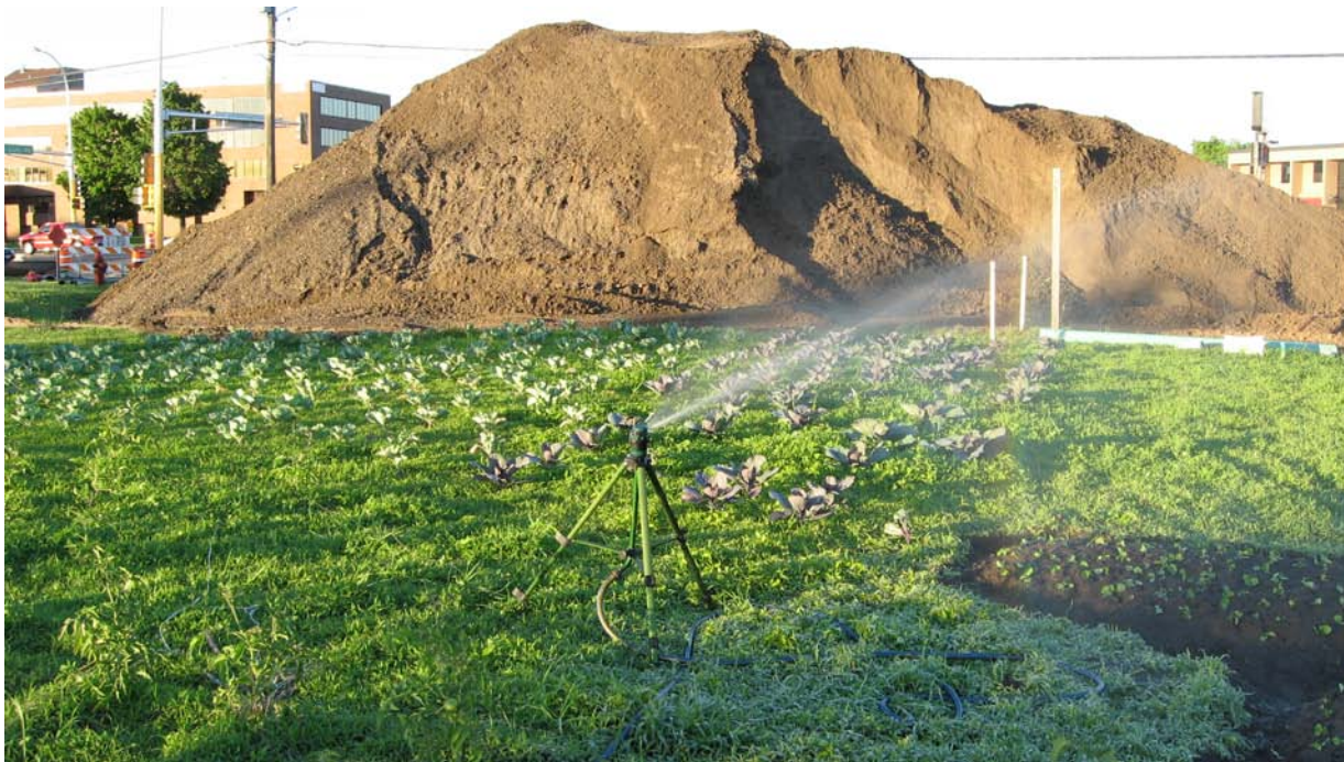
Figure 7. Road construction at Farm site during entire 2010 growing season.
