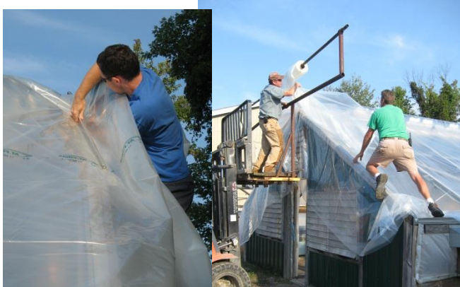
Fig. 1. Replacing plastic on bubble system greenhouse; Canadian expert installing splines (left); UVM and Claussen employees rolling out plastic (right).
