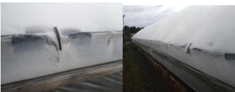
Fig. 4. Black tubing placed vertically between the two layers of plastic, which effectively eliminated the pooling problem.
