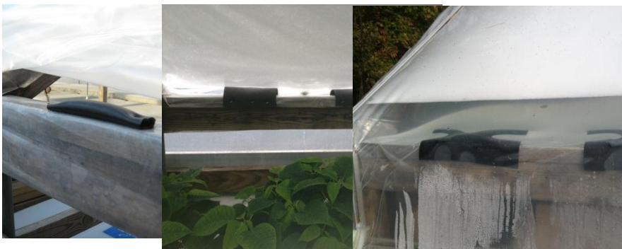
Fig. 3. Device for preventing fluid pooling at the edge of the greenhouse (left to right); black tube attached to hip frame of greenhouse, EPDM plastic covering tube; pooling of the soap solution that continued to occur.
