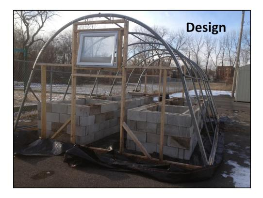
Photo shows uncovered greenhouse in its new location inside a fenced area. You can see the design of the end walls with placement of the window for ventilation and door at the other end.
