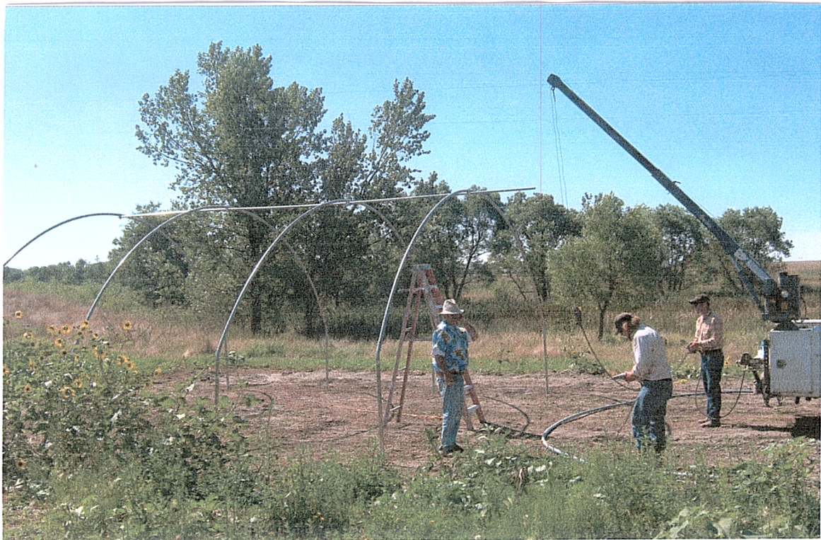
Using the crane on Jimmy's worktruck to set the beams.
