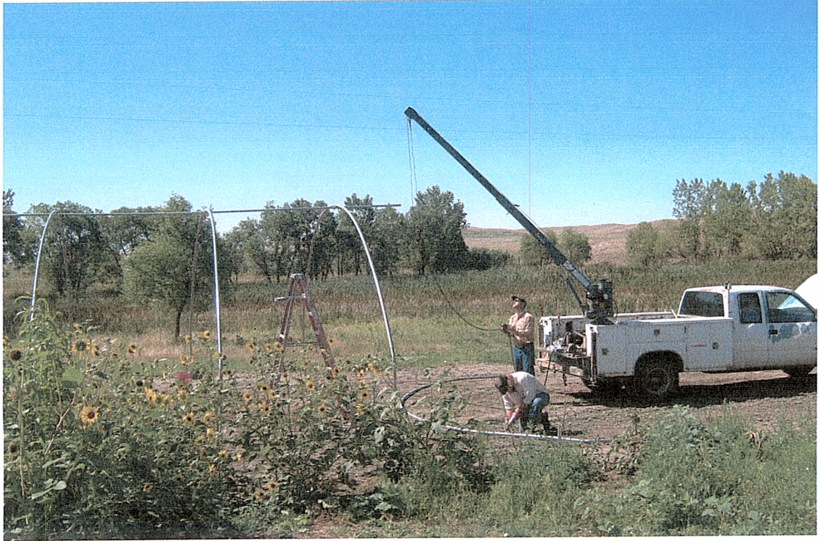
Using the crane on Jimmy's worktruck to set the beams.
