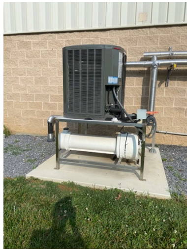
Figure 7. An air-cooled chiller showing a cooling air conditioner unit on top that supplies chilled refrigerant to a cooling loop that flows through coils in an enclosed PVC unit below. Water pumped from the Bio-Organic Filtration tank is cooled as it circulates around the chilled coils and cycled back.
