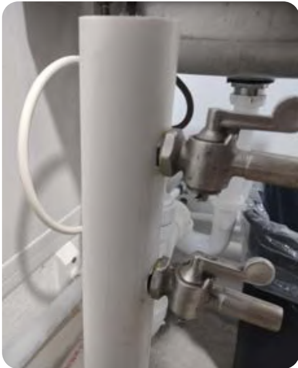
Teflon tape and thread sealant are used to make a air tight seal.
