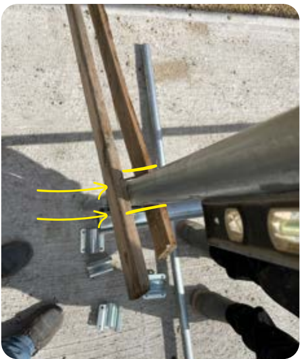
Using the a 3" screw one on either side of the pipe will keep it from falling (3/4" board, 1.5" pipe, 3/4" board = 3"). We used a magnetic level to level the legs prior to securing to bracing.
