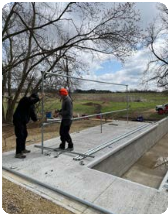
Once vertical, one person can stabilize and the other can attach bracing.
