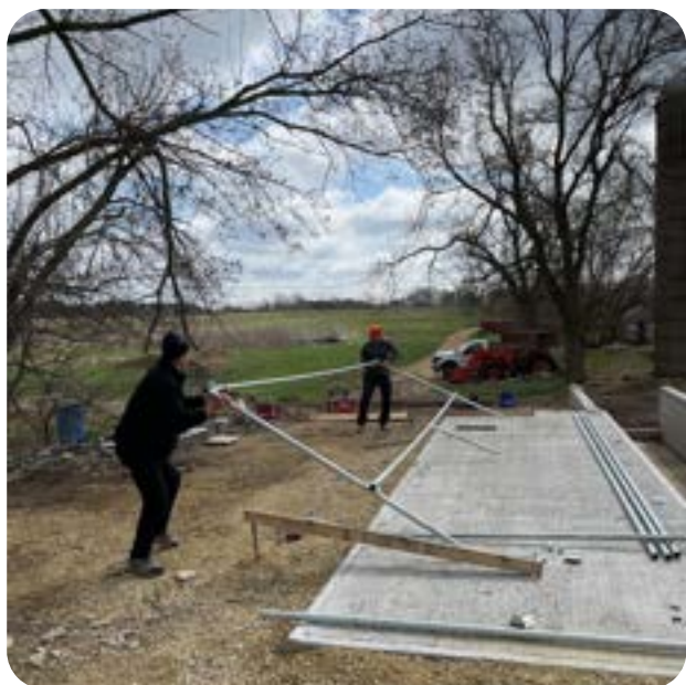
Fittings are tightened down, wall is moved into place and lifted vertical.
