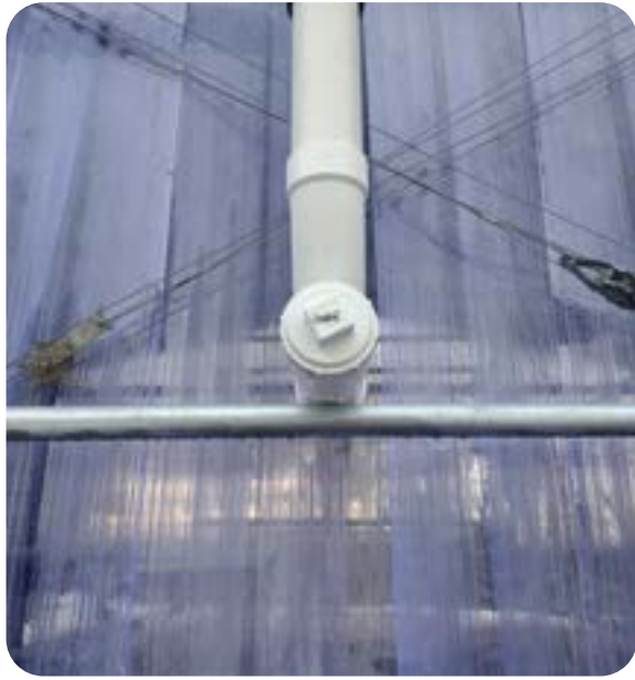
Clean-out fitting and cap for ends of vacuum line for easy cleaning.
