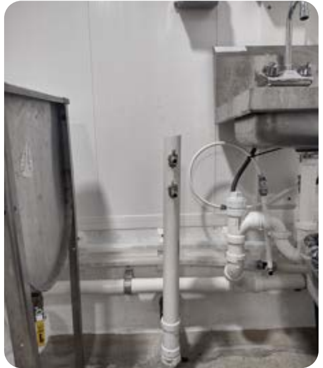
The PVC airline is run inside the milk house using 1.5" pipe and 2 additional stall-cocks are used to operate the Nupulse claw washers. A clean out at the low point allows for draining any water that enters the line.
