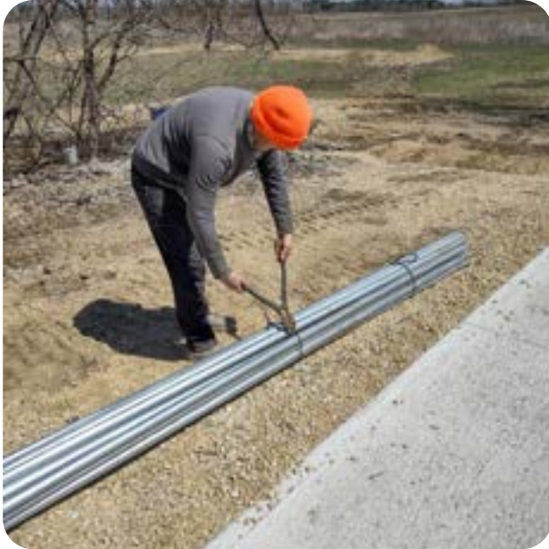
Using bolt cutters to un-band the pipe
