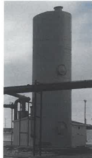
Figure 1. Sunnyside Biological Trickling Filter
