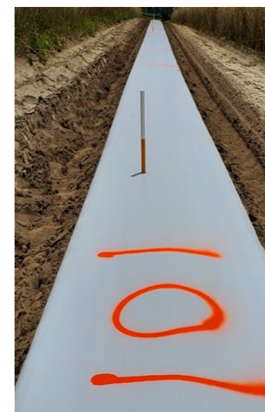
Installation of IRIS tubes
