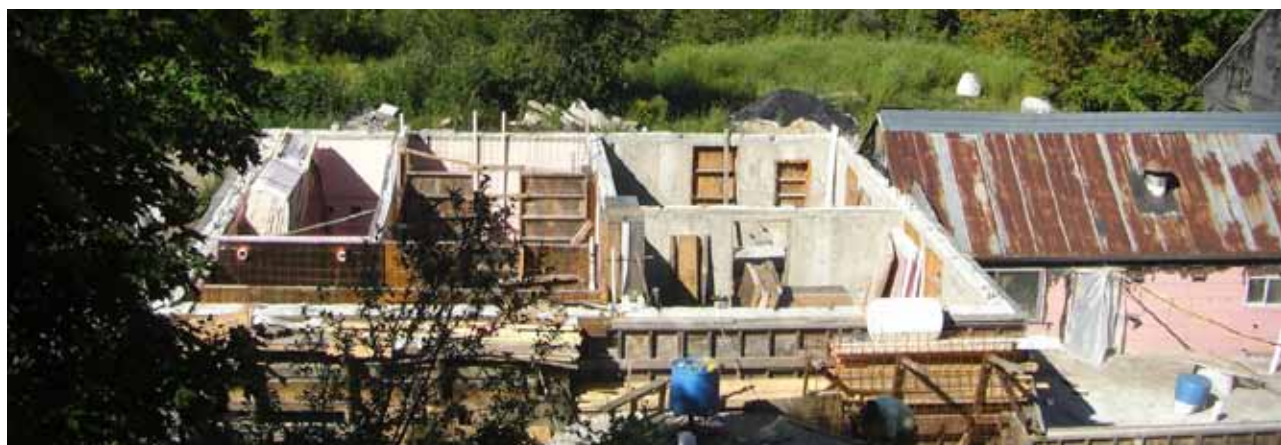
"Butcher Shop Under Construction." Image used with permission of Walter Jeffries. ©2012 Walter Jeffries, SugarMtnFarm.com
