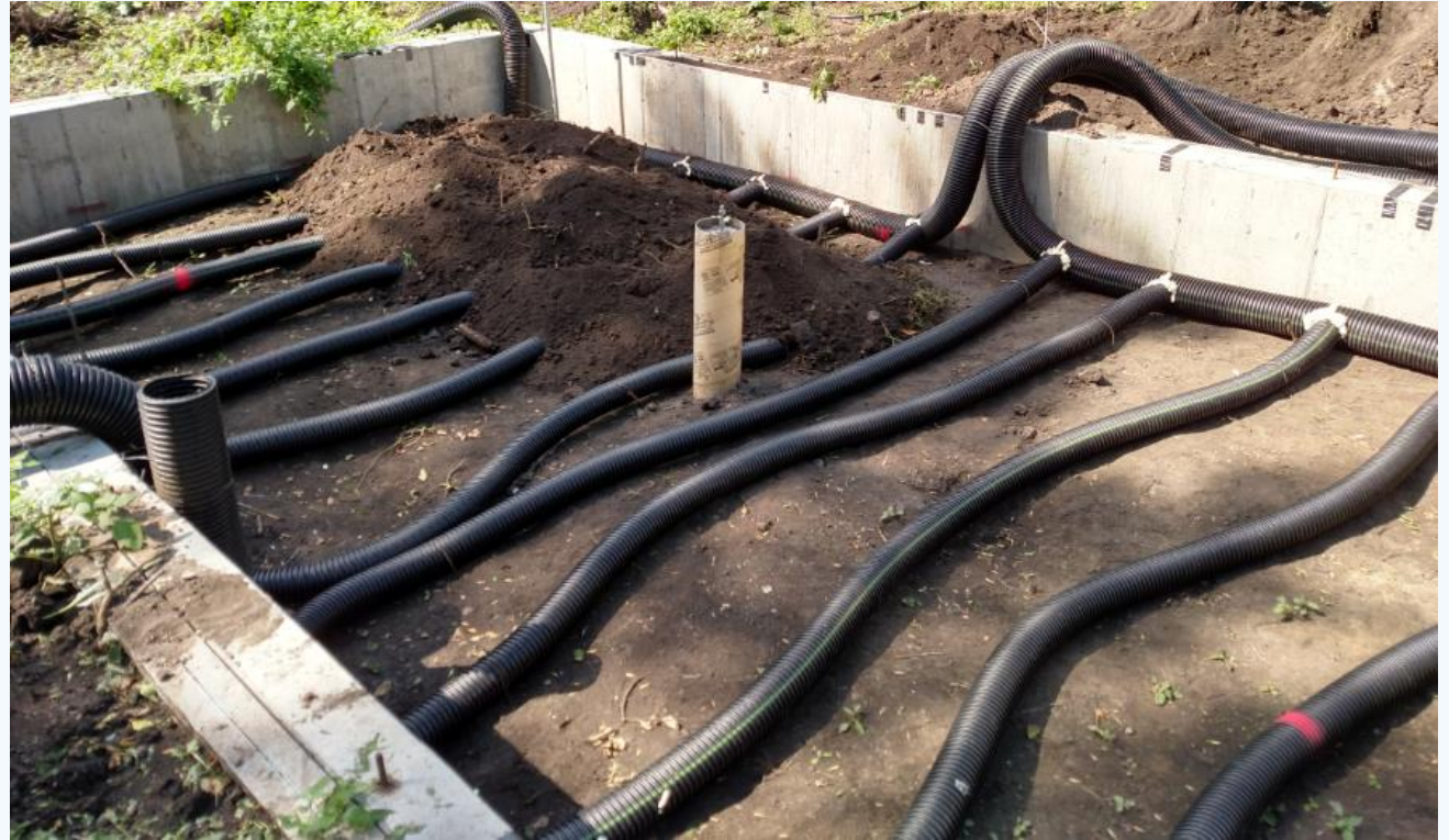
Upper 2ft (0.6m) deep layer of tubes
