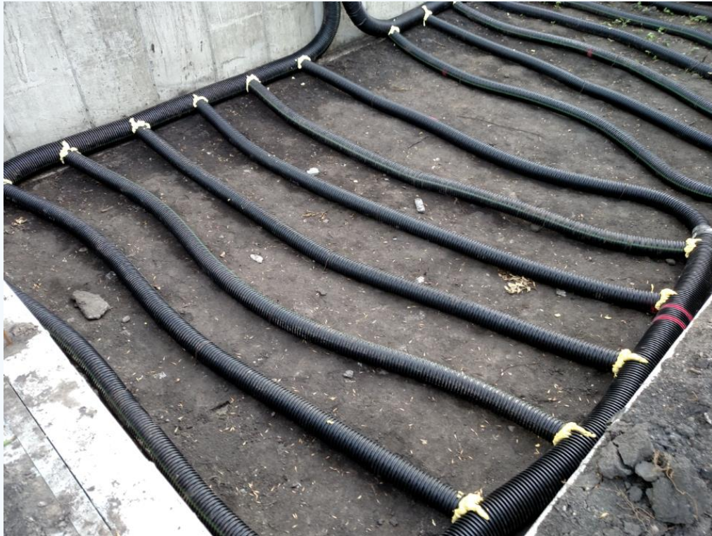
Bottom 4ft(1.2m) deep layer of tubes
