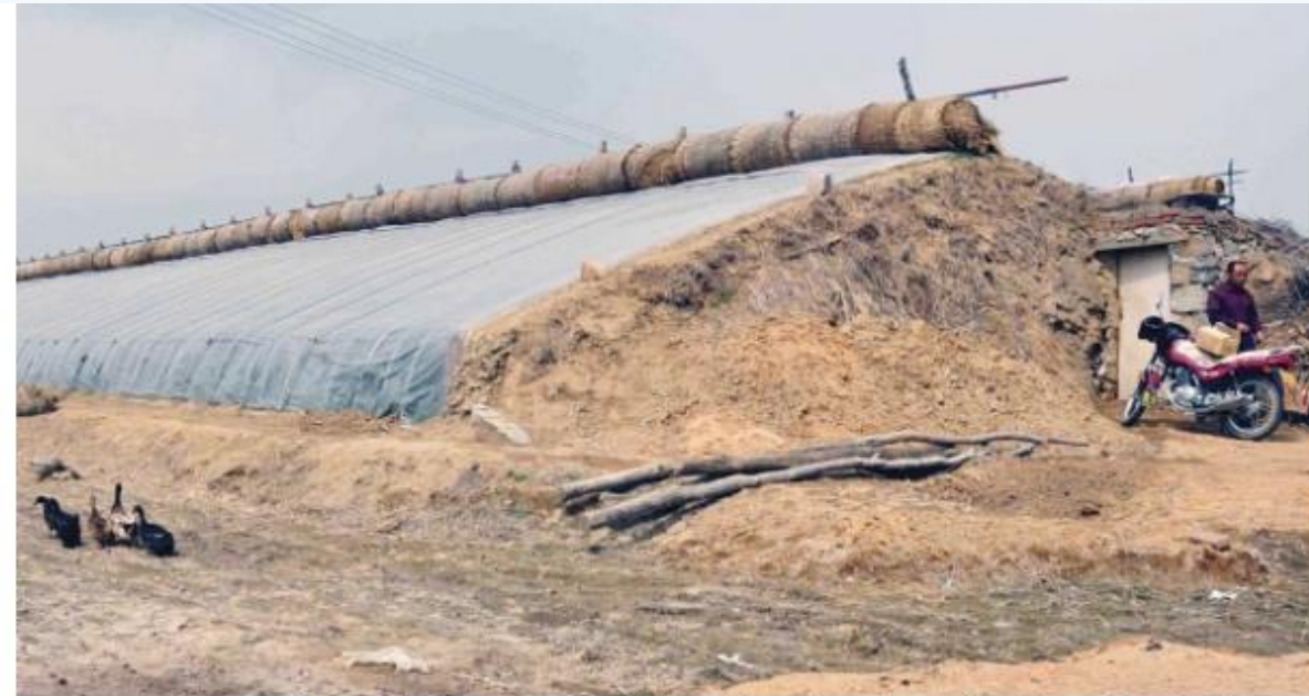
A typical, south-facing solar lean-to greenhouse with sunken floor. The side and back walls are made of earth. Note the nontransparent insulation rolled up at the top of the house. (Courtesy Desmond R. Layne, Ph.D./Washington State University)
