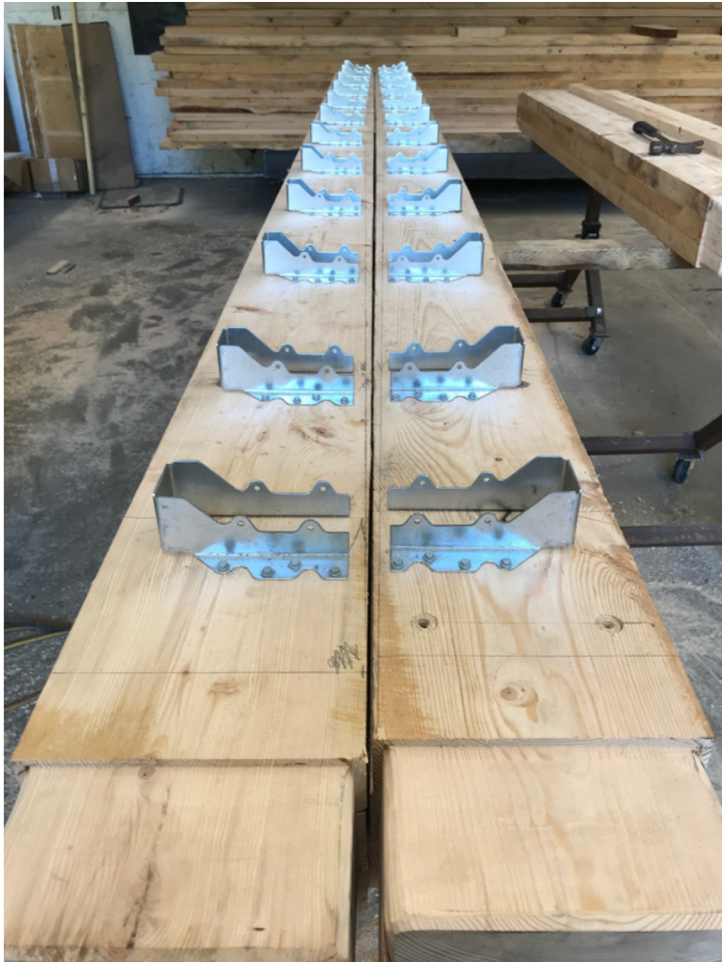
Exact placement of the joist hangers on the inner faces of the floor girders establishes the floor pitch to the central trough drain.
