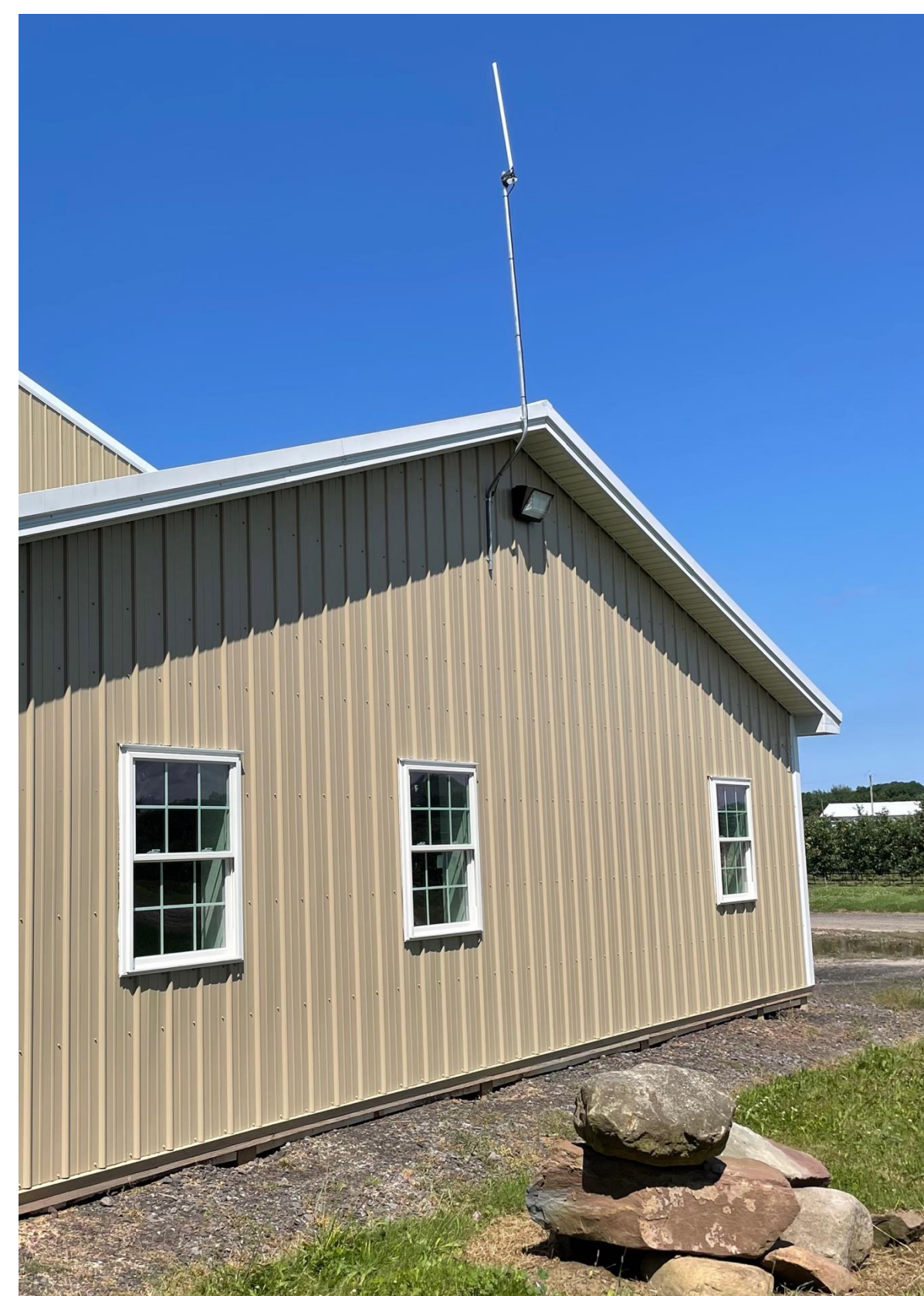
Gateways in fields or on facilities provide LoRaWAN connectivity and pick up LoRaWAN device data
