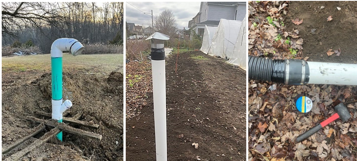
Figure 5: Left: EAHX Intake Riser with wye at ground level and elbows and mesh at intake. Note supporting lumber before backfilling. Center: cone top chimney cap with screen used in other EAHX systems. Right: Corrugated to PVC connection showing tile tape, rubber coupler
