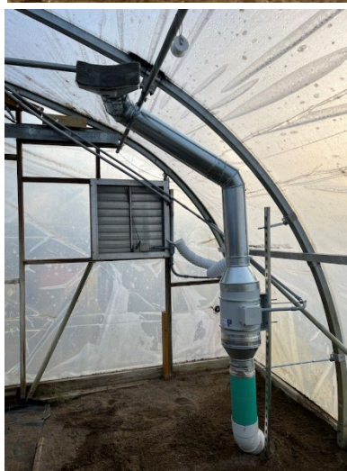
Figure 4 Top: intake and pump access point of EAHX. Bottom: distribution fan for EAHX
