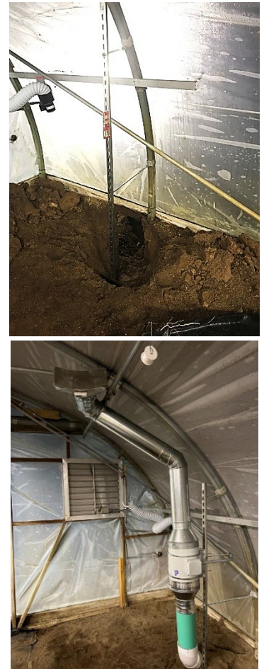
Figure 6 Top: Strut assembly before fan mounting. Note hand-dug trench under high tunnel wall. Bottom: fan and ductwork for air distribution
