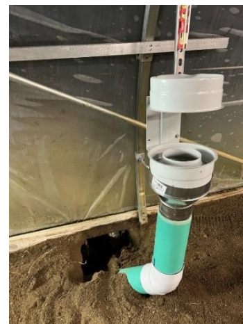
Figure 5 Connecting underground system to fan
