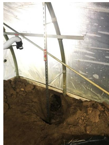
Figure 4 Strut secured to high tunnel with bracket
