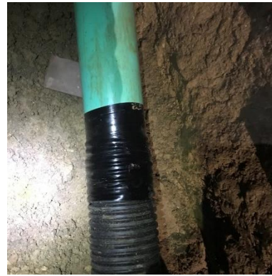
Figure 2 Pipe wrap or 'tile tape' before rubber coupler is slid into place
