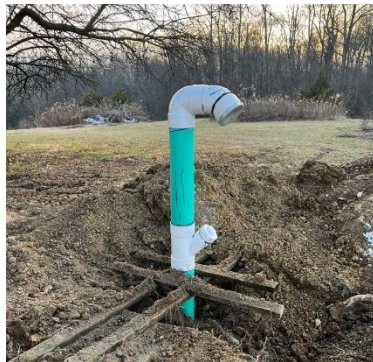
Figure 3 EAHX Intake Riser with wye at ground level and elbows and mesh at intake. Note supporting lumber before backfilling
