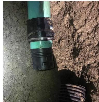
Figure 1 Corrugated connection and flexible coupler
