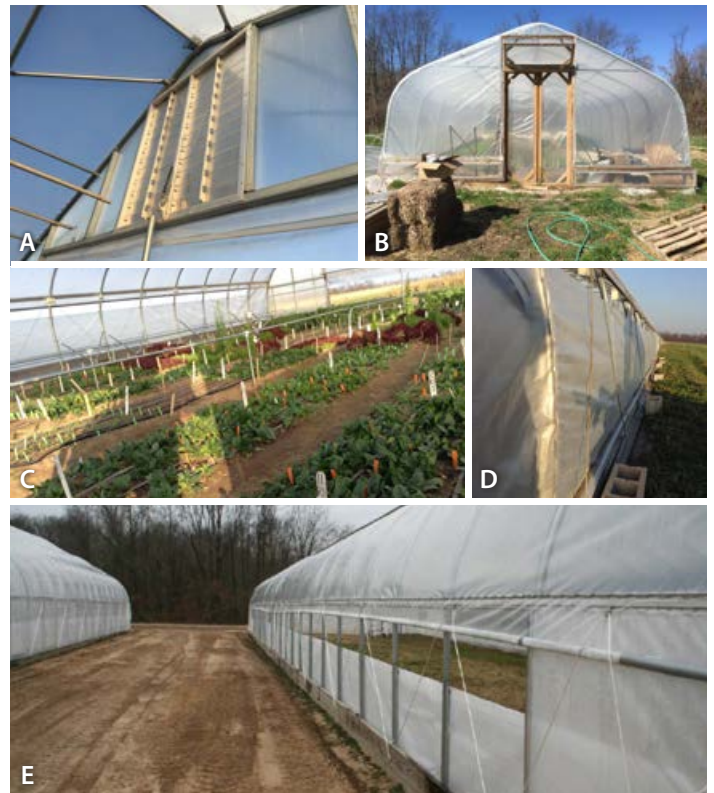
Figure 12. The vents high in the endwall (A and B) and temporary sidewalls (C,D, and E) shown here prevent cold air flowing directly onto low-growing plants. The metal end wall vent shown (A) is operated by a wax-based vent opener. Temporary sidewalls can be removed when temperatures warm. (Photos by E. Bluhm, E.T. Maynard and S. Saha)
