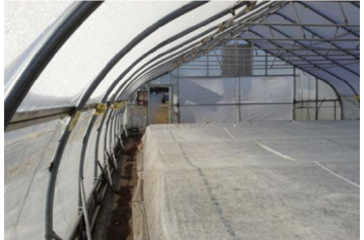
Figure 10. In this structure the side wall lets in more light than the plastic roof in late December because frost and/or snow reduce transmission through the roof plastic. This structure is oriented east-west, with south to the left of the picture, and so the shaded area will remain similar throughout the day as the sun moves across the southern sky. (Photo by E. Maynard)
