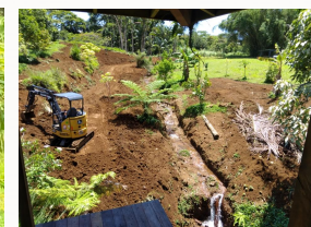
Terracing the steep hillside along the stream banks
