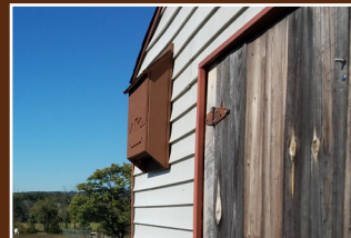
Three-chambered bat house installed on a barn. Photo: Reid Wilbraham
