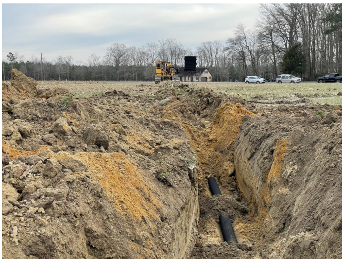
Tile installation at manual drainage water management system in February 2023.
