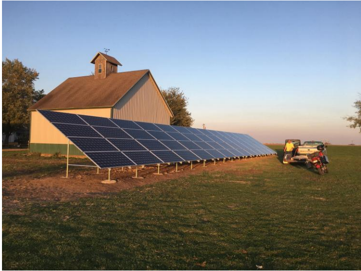
Behind the Meter
