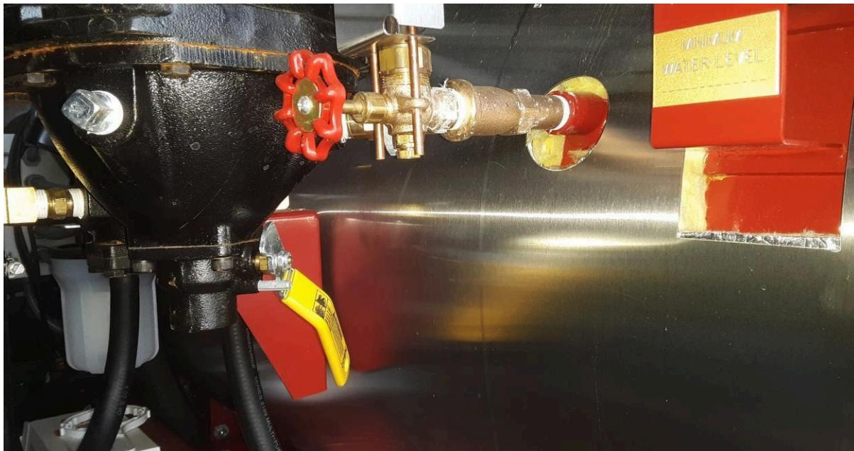
3. If the generator has not been run recently, prime the fuel supply by a few strokes of the plunger that's mounted in the fuel filter.
