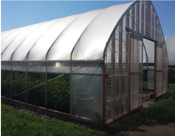
30-foot-by-60 foot high tunnel with roll-up siding for ventilation and temperature management.
