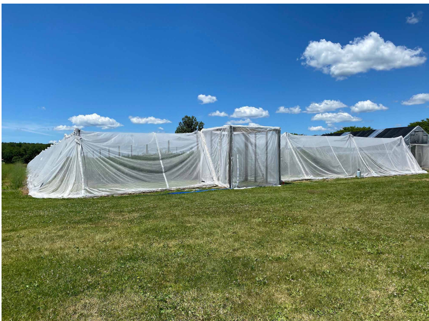
The team's newer support structure and netting system that was erected in 2020.
