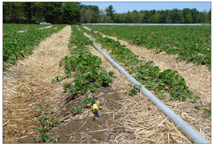
Photo 4-12. Irrigation pipe and risers for providing overhead irrigation for frost protection (D. Handley).
