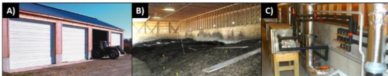
Figure 3.2 Joshua Nelson Energy Recovery Compost Facility located at the University of New Hampshire Burley-Demeritt Organic Dairy Research Farm in Lee, New Hampshire, USA. The images show A) the exterior doors to the facility where compost feedstock is loaded, B) piles of composting material in the facility, and C) the back of the facility where the gas exhaust from the facility is piped, allowing for heat recovery and measurements.
