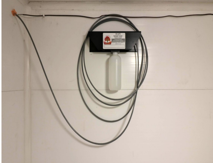
▲ The DewRight Humidity sensor accurately measures and reports the relative humidity to a computer which controls humidifiers to optimize storage conditions to ideal set points for storage crops.
