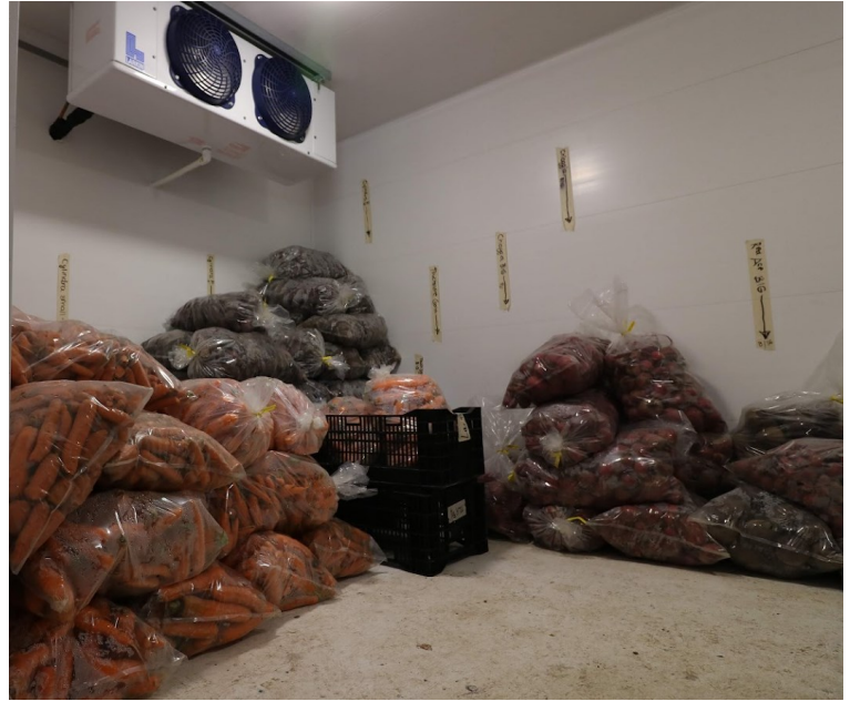
▲ This cooler is equipped with a commercial split refrigeration system and used when there needs to be a lot of field heat removed quickly. Shelves are planned, but temporary organization is accomplished with masking tape.
