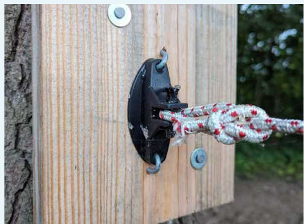
Note the wide washers. Those are essential! If you don't include those, the nail will pull through the board, undoing your work. Also, consider using long-lasting boards while you're at it.
