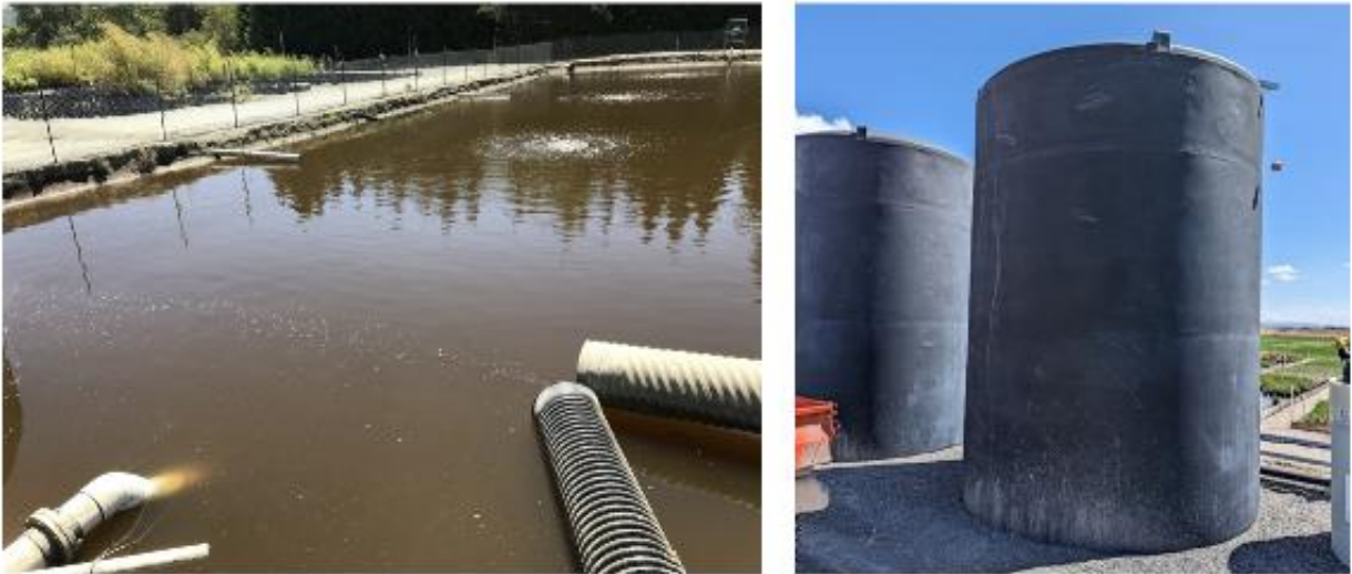
Figure 1: Retention pond (left) and above ground storage tank (right) to collect Irrigation return flow in nursery.
