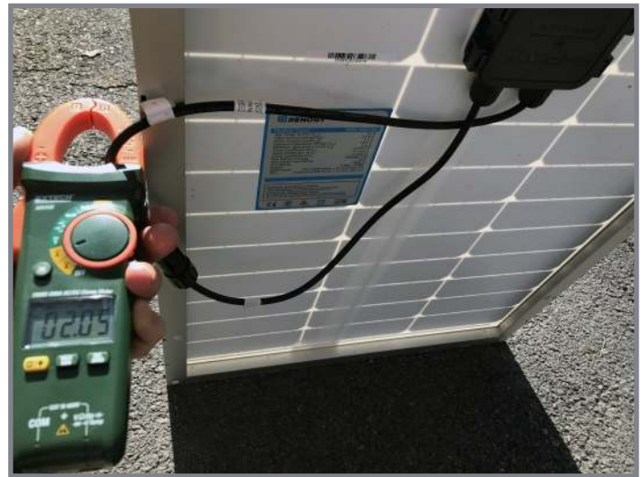
Figure 6. The short-circuit current ( I_{sc} ) of a 50 watt solar module is measured using a digital clamp-on multimeter which encloses one of the conductor leads from the solar module. With the positive and negative leads of the solar module connected to each other, a current of 2.05 A is measured during less than full sun conditions.
