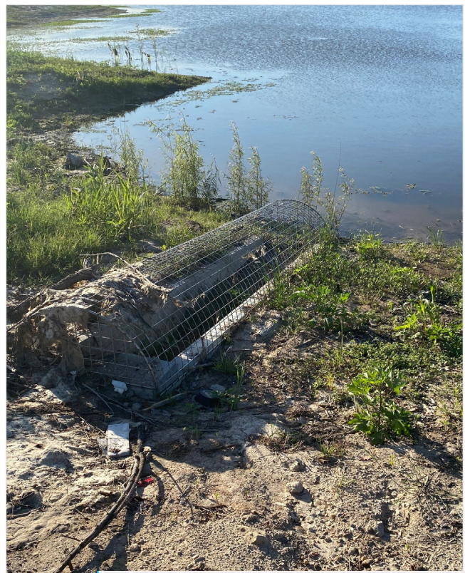
Figure 9. A pond spillway demonstrating a grass carp escapement barrier to prevent unintended release of triploid grass carp to the wild.
