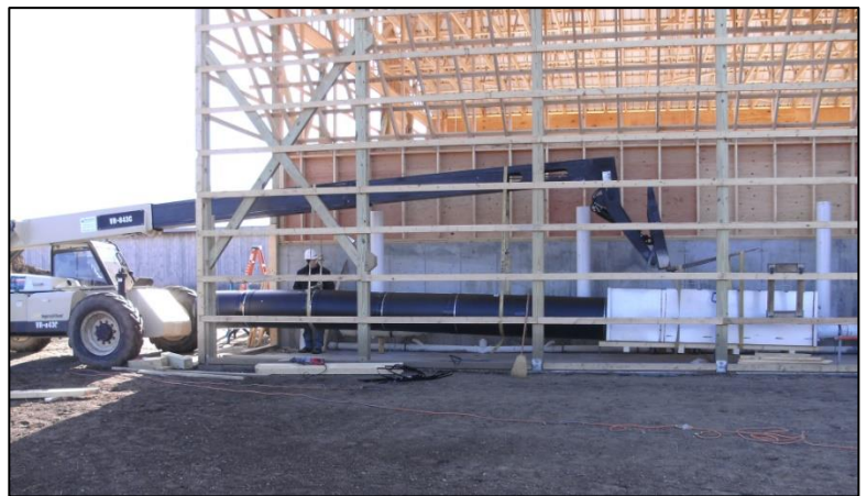
Figure 48: Delivery of Agrilab Technologies Heat Exchange Unit
