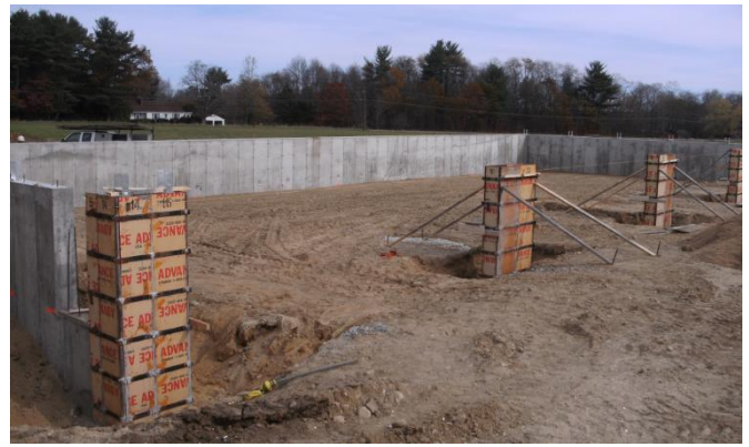
Figure 14: Concrete Piers at the UNH Composting Facility
