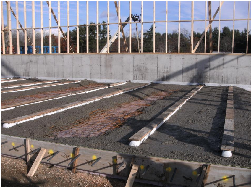
Figure 30: Concrete Pour for Main Composting Floor
