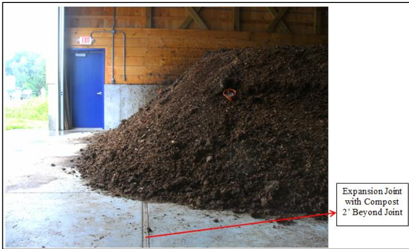
Figure 23: Expansion Joint Between Compost Floor and External Apron
