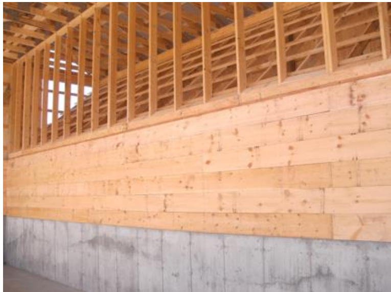
Figure 17: Back Push Wall at UNH Composting Facility
