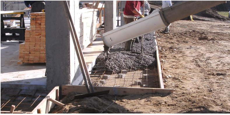
Figure 39: Specifications when Pouring the External Concrete Pad
