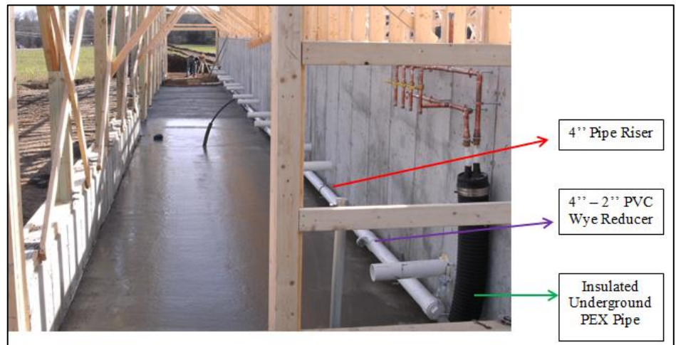
Figure 40: Specifications when Pouring Back Mechanical Floor
