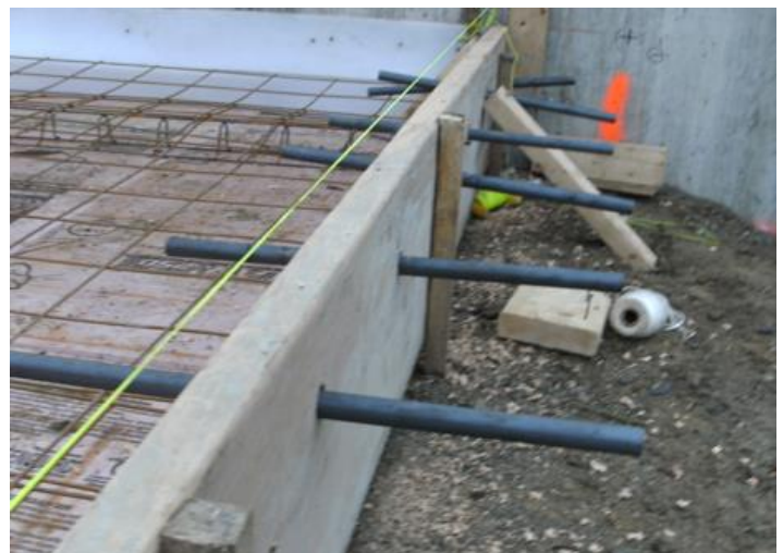
Figure 22: Concrete Slab-Connecting Dowels at UNH Composting Facility
