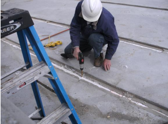
Figure 32: Drilling of Aeration Holes
