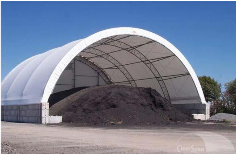
Figure 19: High-Tension Fabric Structure with Waste Block Walls (ClearSpan 2013)
