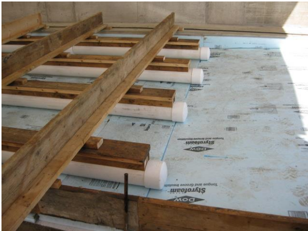
Figure 27: Alternate Cover Plate Form Setup
