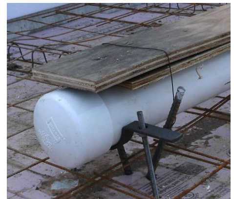
Figure 26: Aeration Line Forms for Cover Plates
