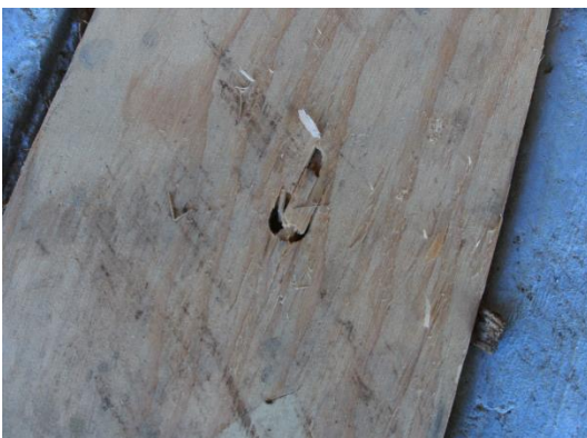
Figure 37: Aeration Hole with Chipping
