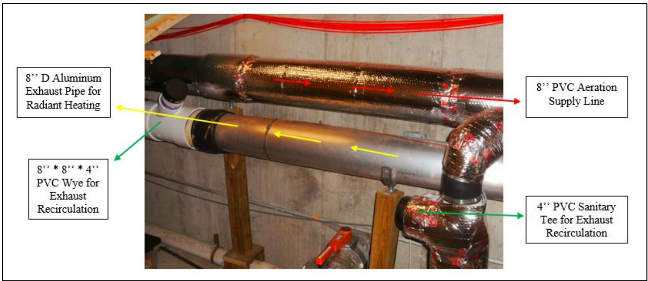
Figure 44: Exhaust Vapor Recirculation Connection Points
