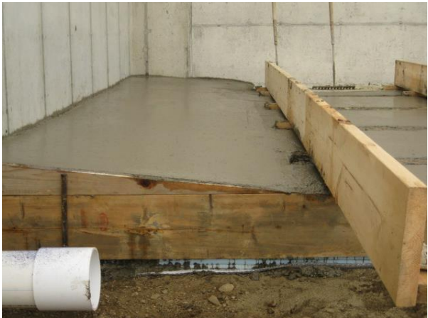
Figure 28: Alternate Cover Plate Form Setup
