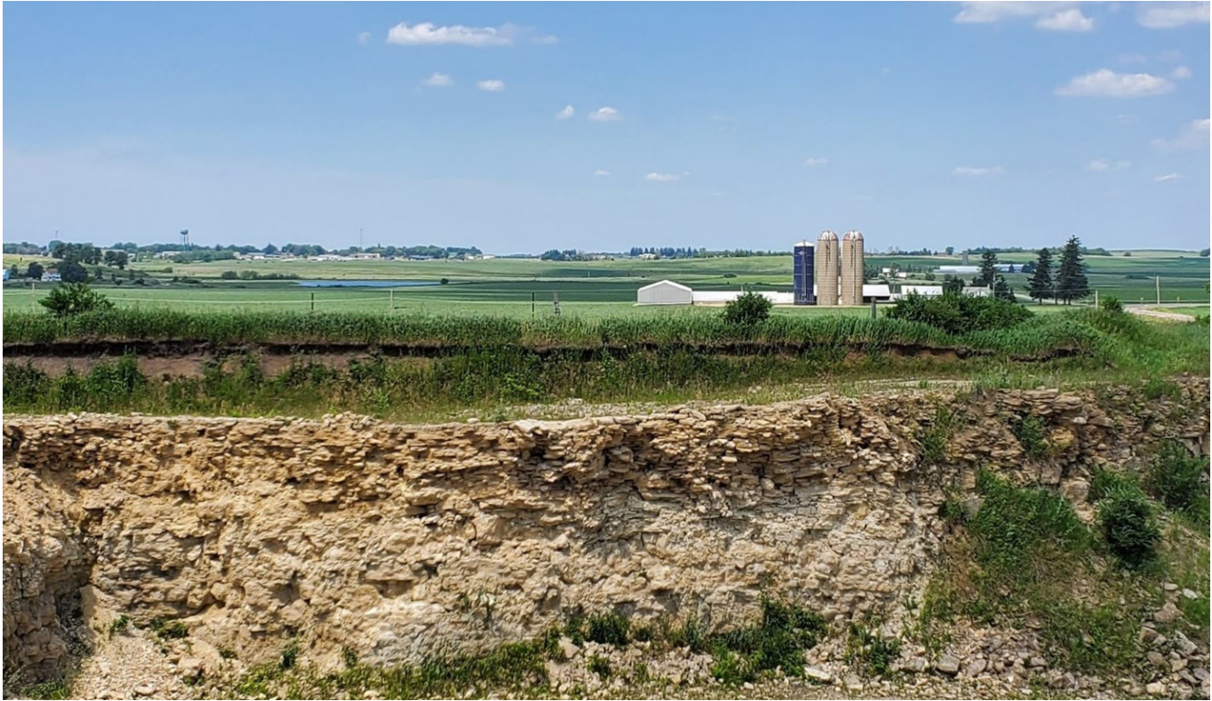
Figure 3. Diagram of preferential flow and shallow depth to bedrock to illustrate greater leaching risk Photo: F. Arriaga
