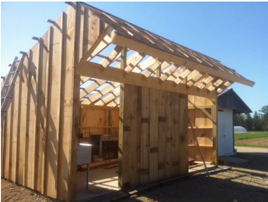
(partially finished packing shed at King Hill Farm )
