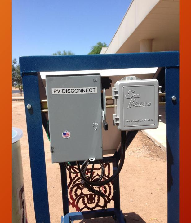
We learned other safety tips like using a locking electric connection case to control a connection either being made or disconnected at the wrong time
