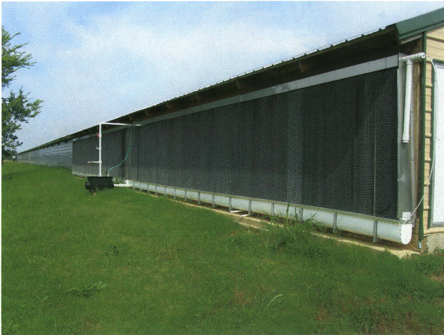
Cooling pads of tunnel-ventilated poultry production structure.
