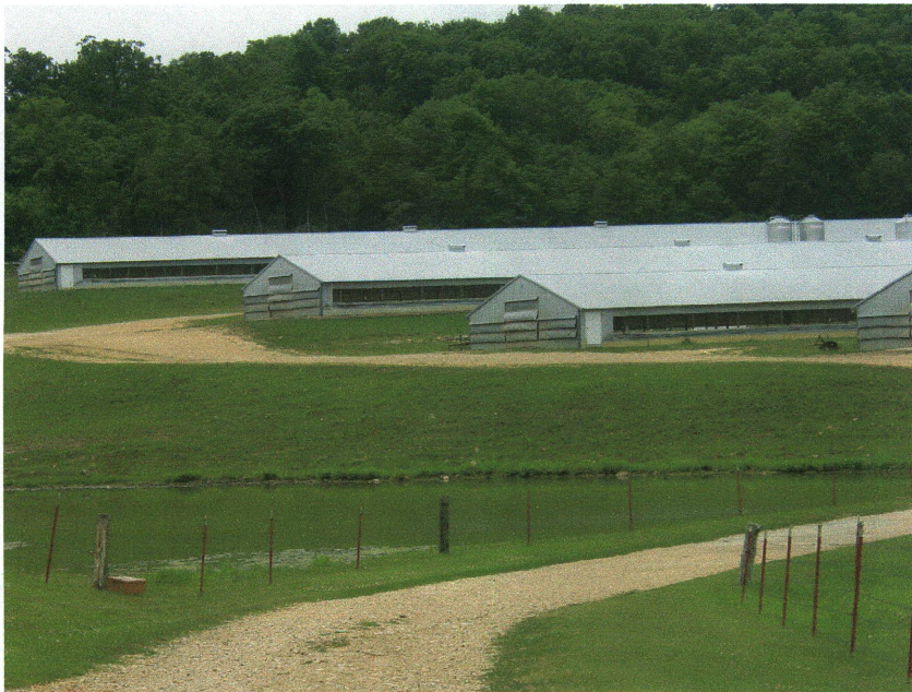
Poultry operation in Arkansas using positive pressure cooling and drop walls.
