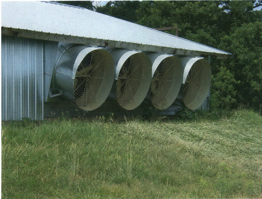
Exhaust fans of tunnel-ventilated poultry production structure.
