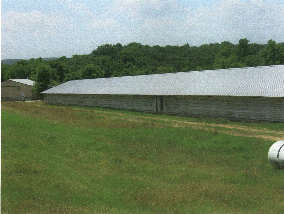
Exterior of standard steel-framed drop-wall poultry production house.
