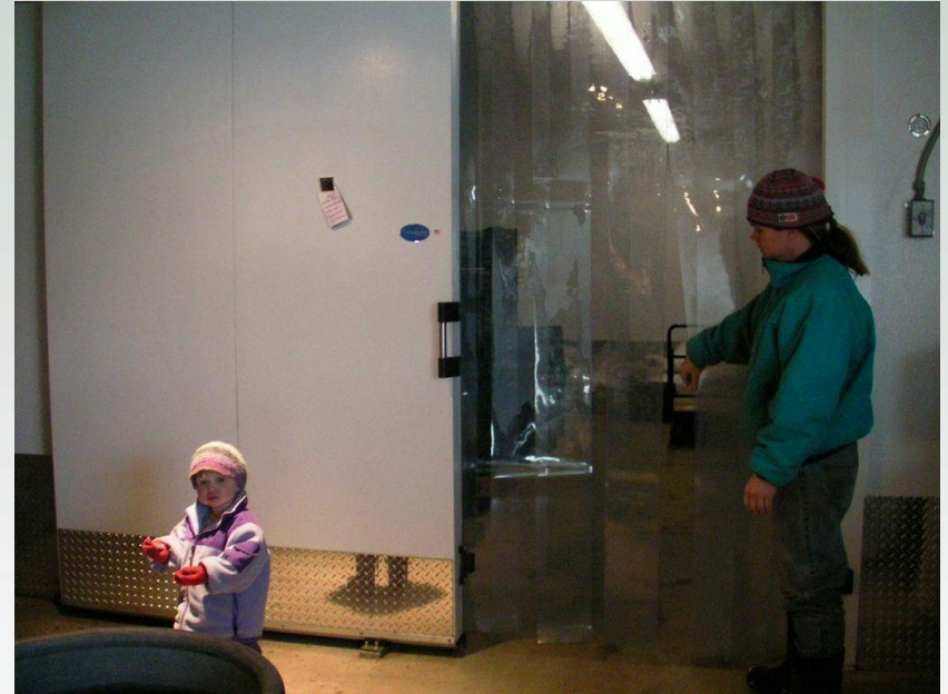
Sliding cooler door with plastic curtains at Jericho Settlers Farm
