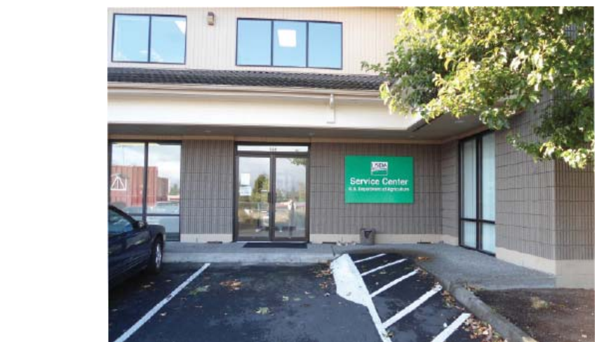
Below is the present site, on a third corner across from Jack in the Box.
