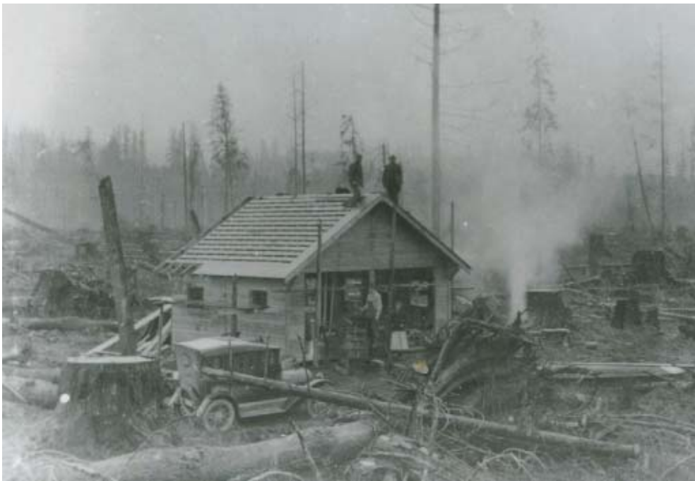
Building the garage on the Tillman Farm.
