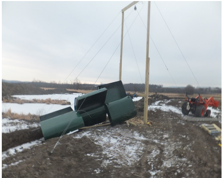
The tower is already anchored in place. The rotor assembly is in position and ready to be raised. The tractor, visible on the right, lifts the half-ton unit into place.
