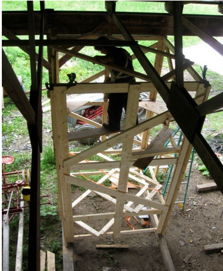
Building the prototype tower under our pole barn.
