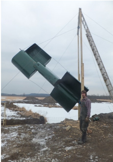
With the bottom of the shaft anchored to the lower cross beam, the rotor was raised into position with a cable pulled by a tractor, threaded through a pulley on the top beam.
