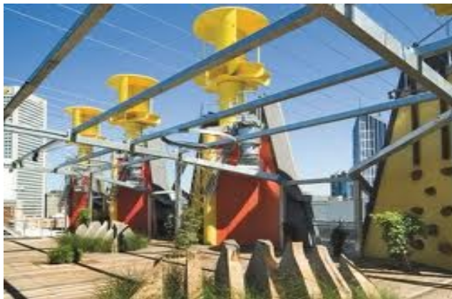
Above: Yellow Savonius rotors grace the skyline of Melbourne, Australia. They are part of a comprehensively-designed energy-conserving office building.
