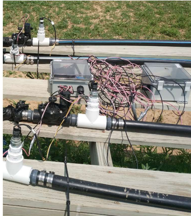
Connect to valves and pressure sensors
