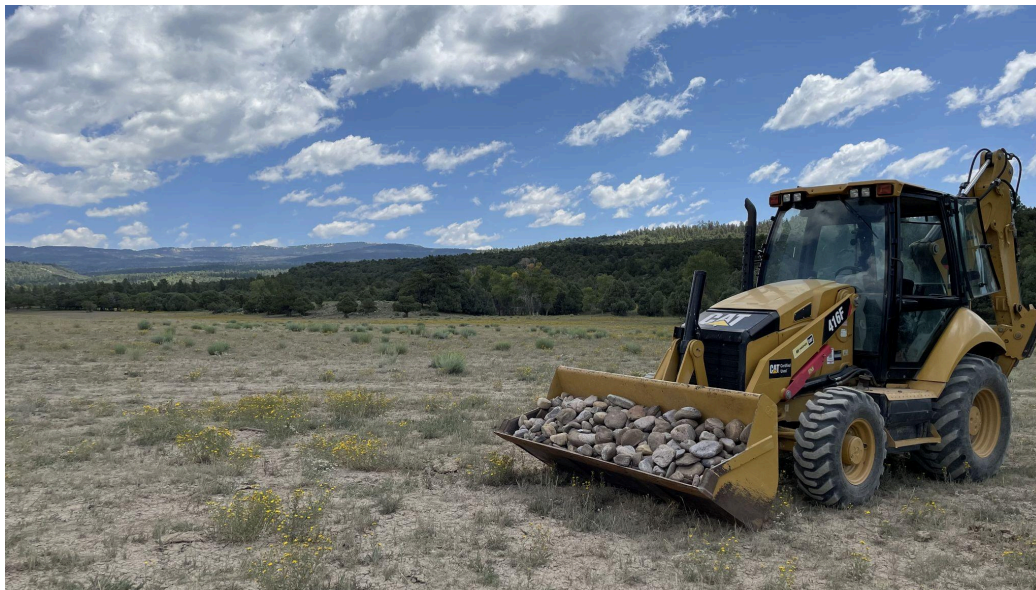
Figure 6: Backhoe transporting rocks to sites
