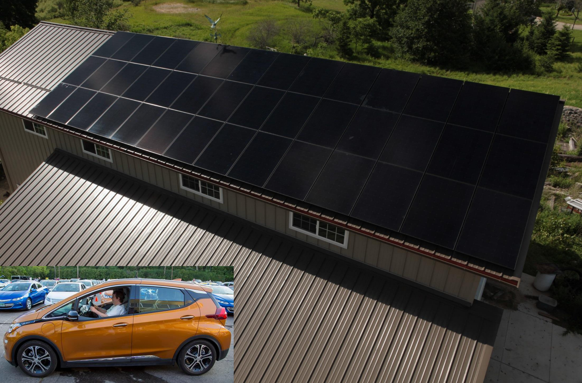
14.1 kW of solar panels and a 2017 Bolt EV
