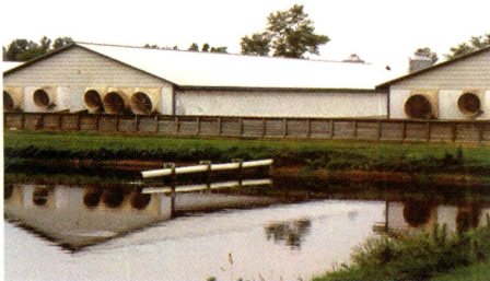
A lined earthen basin is an appropriate storage structure for liquid manure.
