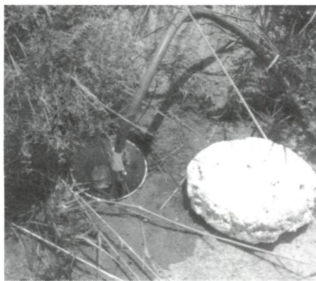
Barker used 8-inch schedule 20 PVC for a casing around each underground coupler.
